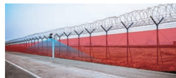
Airports Perimeter Security
